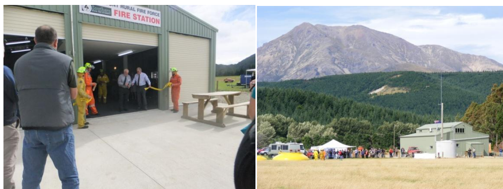
Photo: Blackmount VRFF fire depot official opening February 2011
