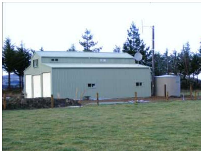
Photo: Blackmount VRFF fire depot construction as at August 2010
